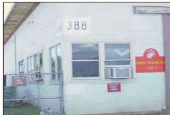
Window additions and air-conditioning units in the northwest corner of Facility 388
