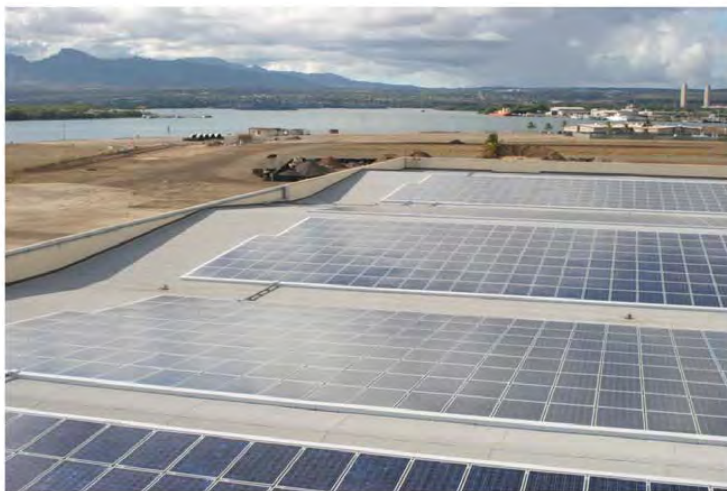
Enclosure 4. Example of surface laid PV system similar to PV system proposed for Hangars 101, 102, 103, and 104 aboard MCB Hawaii.
