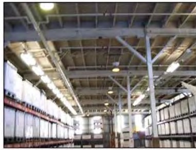
Interior of Facility 270 showing tongue and groove ceiling /roof decking.
