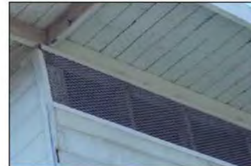
Vent below eave at Facility 388.
