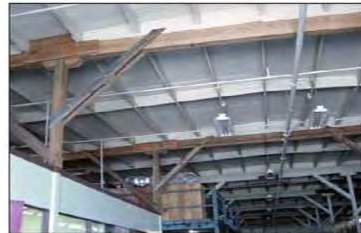
Repaired truss system inside Facility 388. Note added pipes for sprinkler system.
