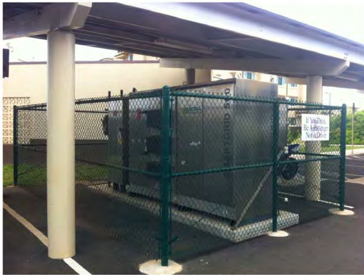
Enclosure 3. An example of an inverter on base.
