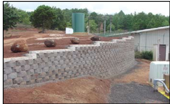
Erosion Control at Mākaha Ridge Tracking Station
