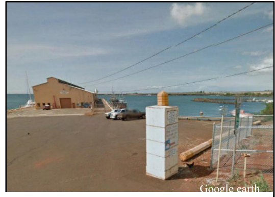
View of building and pier at Port Allen
